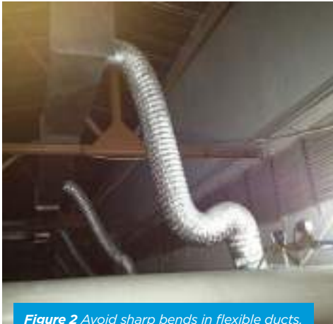
Figure 2 Avoid sharp bends in flexible ducts.
