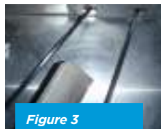
Figure 3 Worn fan belt.
